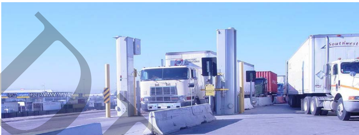
Figure E-3. Empty Truck Portal Towers
